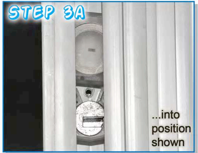
Locate balance assembly in jamb
